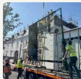
Glazing Refurbishments Ltd (Army, West Midlands)
